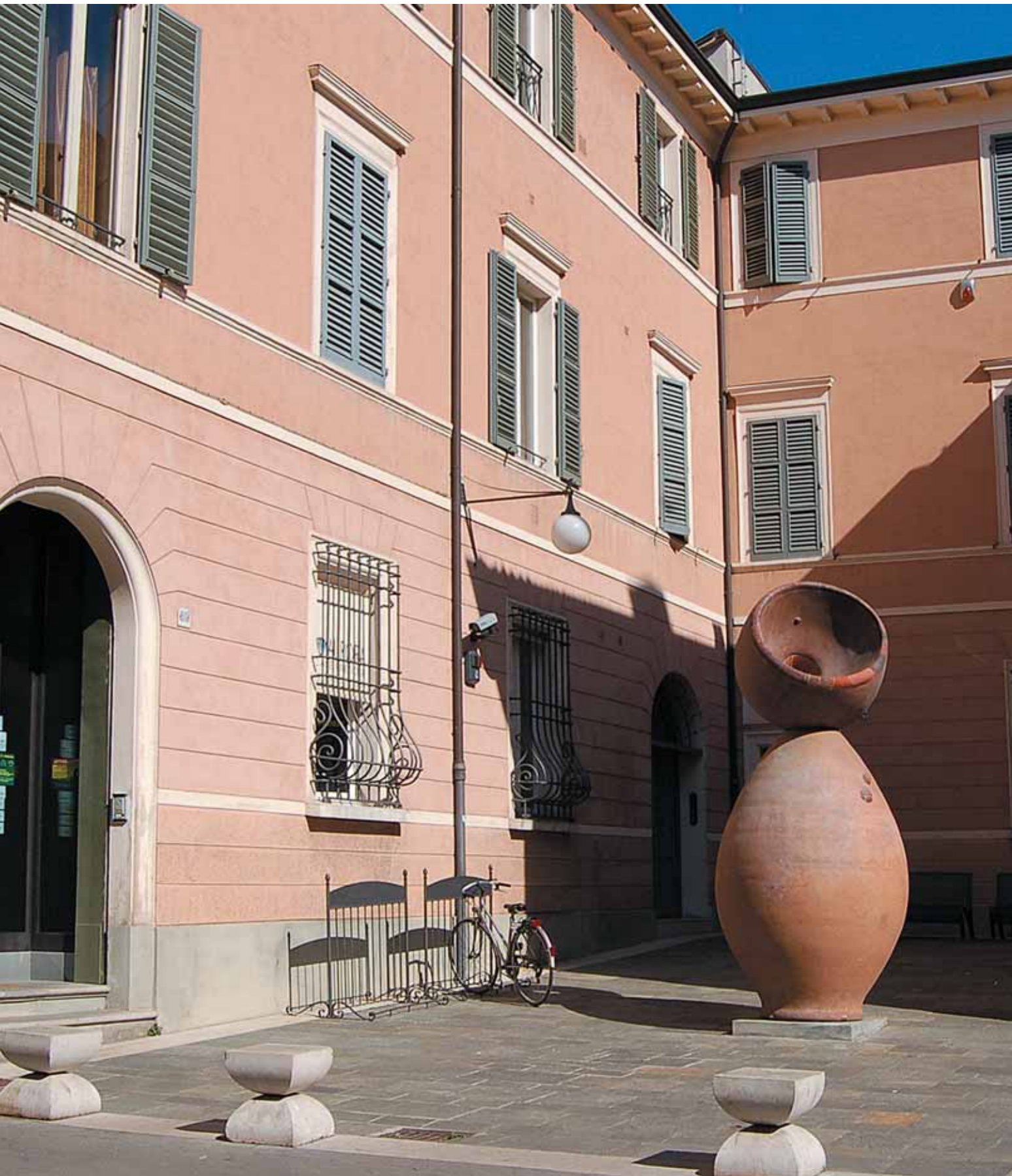
Small square next to the Chiesa del Suffragio church. A corner that was once covered in asphalt is restored to a more suitable appearance, featuring a balanced dialogue between old and new. The stone Lucerne flooring and contemporary posts in travertine stone frame the most important and most beautiful ceramic sculpture in the centre, the work of international artist Franz Stabler (2000).
