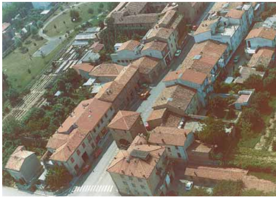
Top, the anomalous situation of the present day in which the Gateway has been conceived as an isolated element to be emphasised: an intervention which can be attributed to a mistaken conception of historical restoration.
